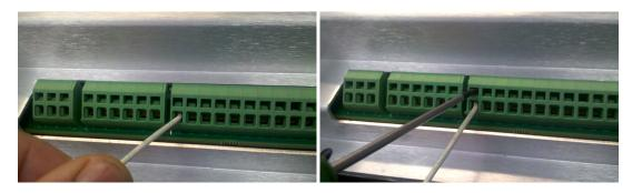
Figure 2-1. Installation of Wiring into Terminal
